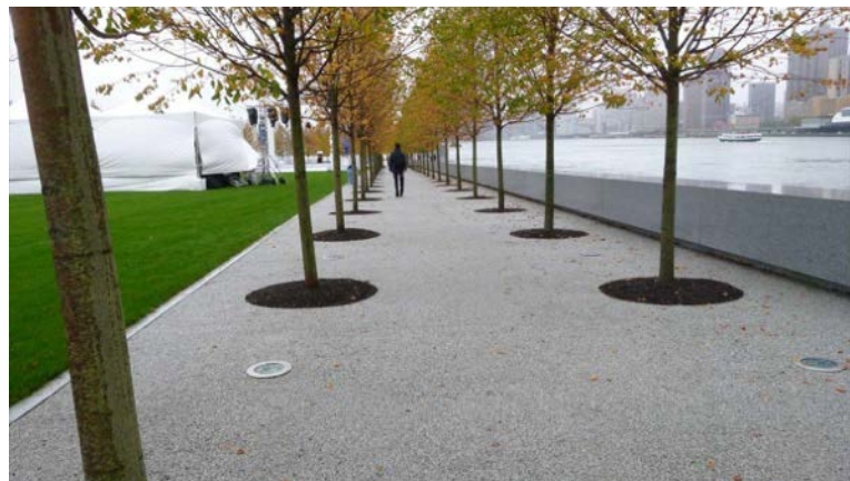
Permeable Resin-Bound Surfaces: Eco-friendly tree surrounds using porous materials. Allows water penetration, supports tree health, and provides a smooth, accessible surface. Ideal for urban settings, combining sustainability with ADA compliance.
